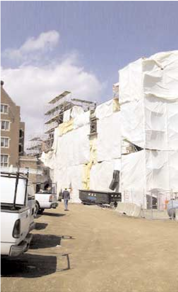
Taft: (left and top right) Thanks to the mild weather and the extensive use of shrouding over scaffolding, as shown in these two views, O&G crews made steady progress through the winter on exterior masonry at the Taft School. The typical expenses associated with heating a project through the winter were also cut considerably by warmer temperatures and the scaffold enclosures. (right) Architectural details abound: Project Manager Jason Travelstead, standing in front of some of the energy-efficient, single-pane English windows that feature lead divisions to match the school's existing fenestration.
