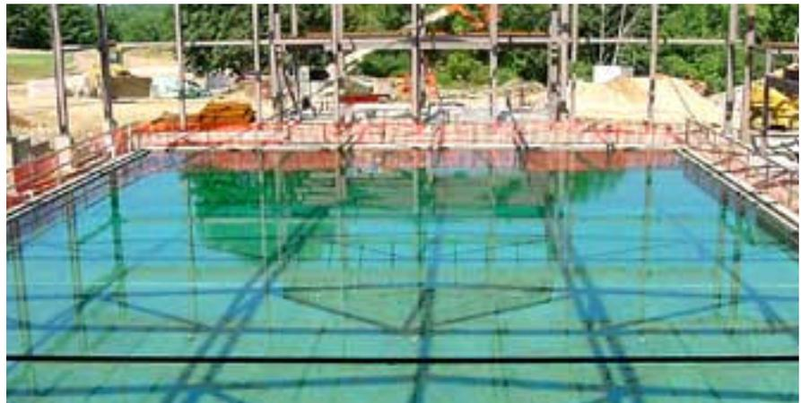
**Hotchkiss School gets a new natatorium:** *In Lakeville, CT, O&G crews are building Hotchkiss' new indoor swimming pool. (top) Workers frame in the structure, seen to the left; (bottom) the concrete pool in the middle of its three-day water test for structural integrity.*
